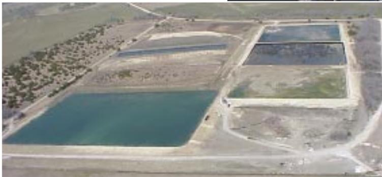
**LEFT:** Three multipurpose soil cells were constructed in 2001 to address perchlorate-contaminated soil and source area groundwater in Area M. The soil cells enabled anaerobic soil treatment while allowing carbon and nutrient-rich water to infiltrate into the perchlorate-contaminated aquifer.
