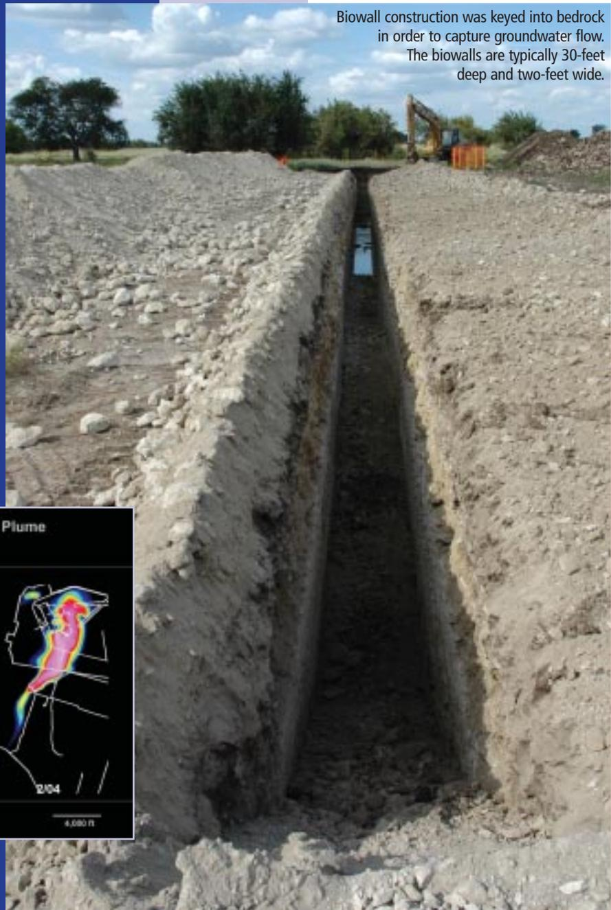
Biowall construction was keyed into bedrock in order to capture groundwater flow. The biowalls are typically 30-feet deep and two-feet wide.
