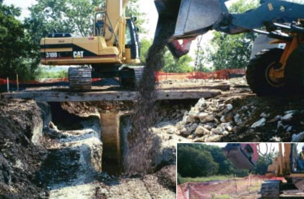
The biowalls were excavated with a hydraulic excavator (shallow trenches) or rock-trencher (deep trenches) and backfilled with a mixture of mushroom compost, pine wood chips, soybean oil, and limestone aggregate. Diffuser pipes were installed on the bottom of each trench to allow for future injections of soybean oil or other carbon substrates as needed.
