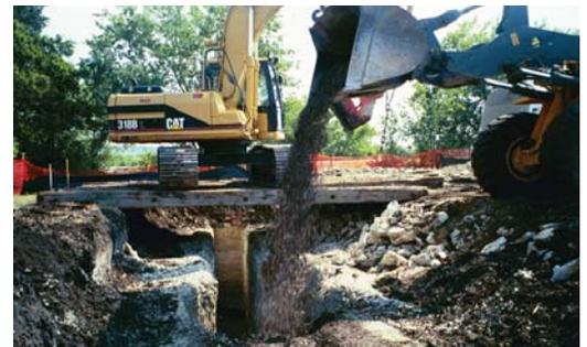
*Media Backfilling of Biowall Trench*
